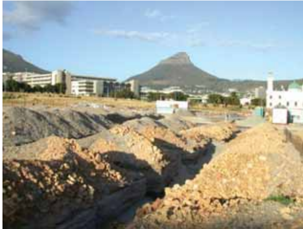
Digging of foundations for the Pilot Project
