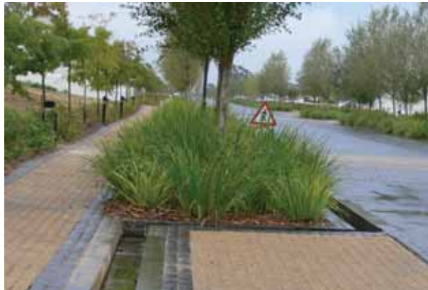
Bio swales and channels can be integrated into the urban landscape and help attenuate and clean storm water
