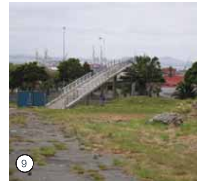
The pedestrian foot bridge(s) over the freeway
