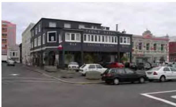
Photo from the East City illustrating the low scale historic nature of this part of the city with typical heights ranging from 2-6 storeys
